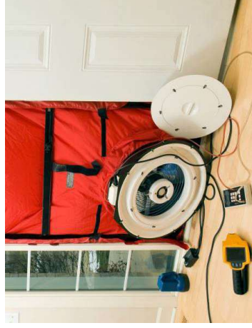
Above: A blower door test can be an effective way to reveal air leaks in buildings.
