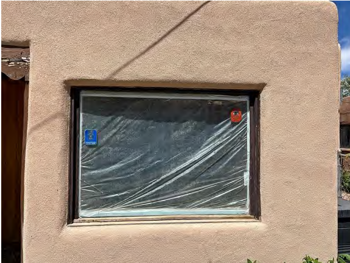
Photo 5: Window at entry vestibule. Camera facing west.
