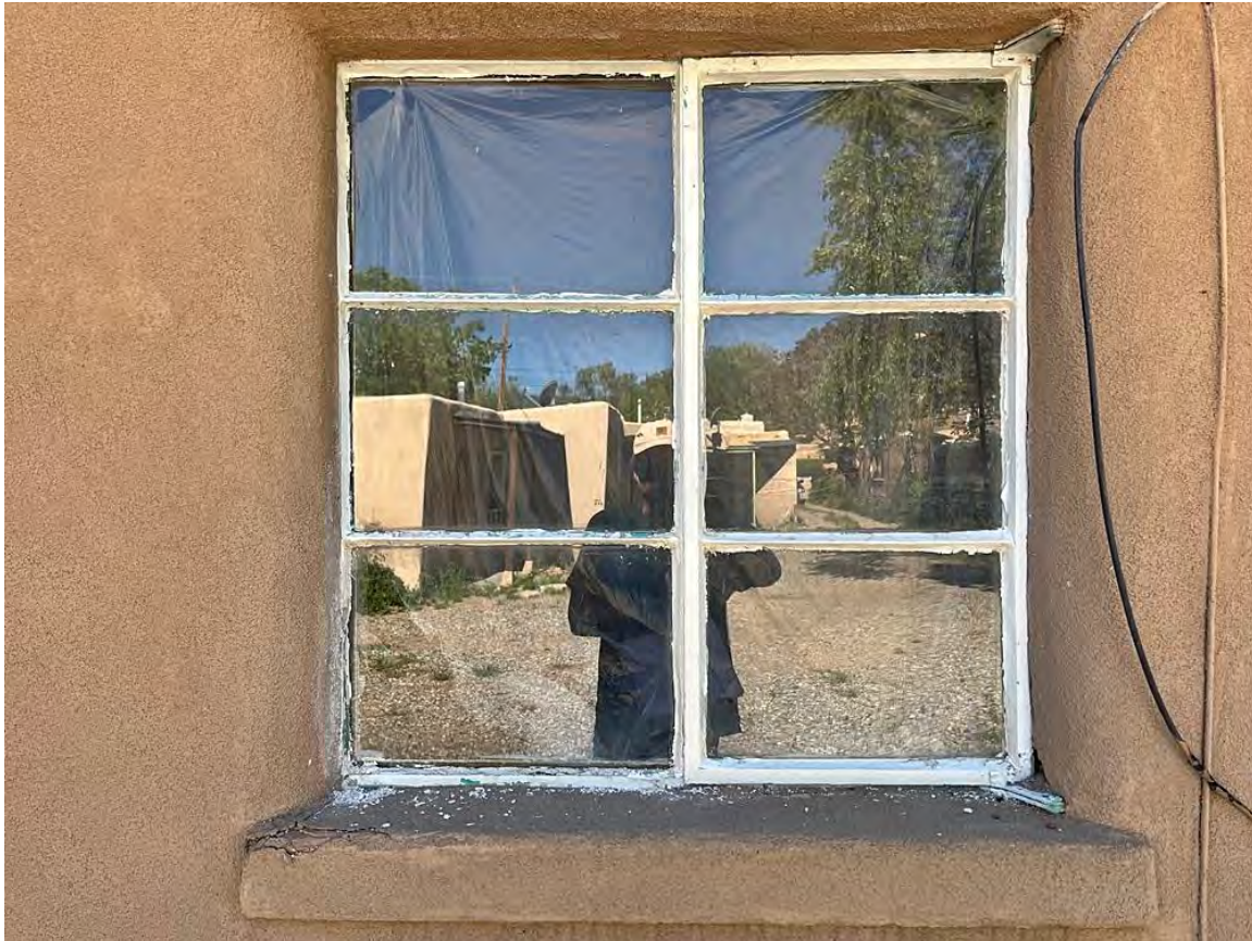
Photo 34: Camera north of entry. Camera facing west.
