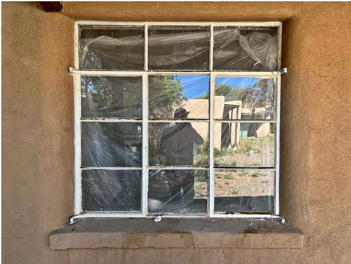
Photo 33: Window south of entry. Camera facing west.
