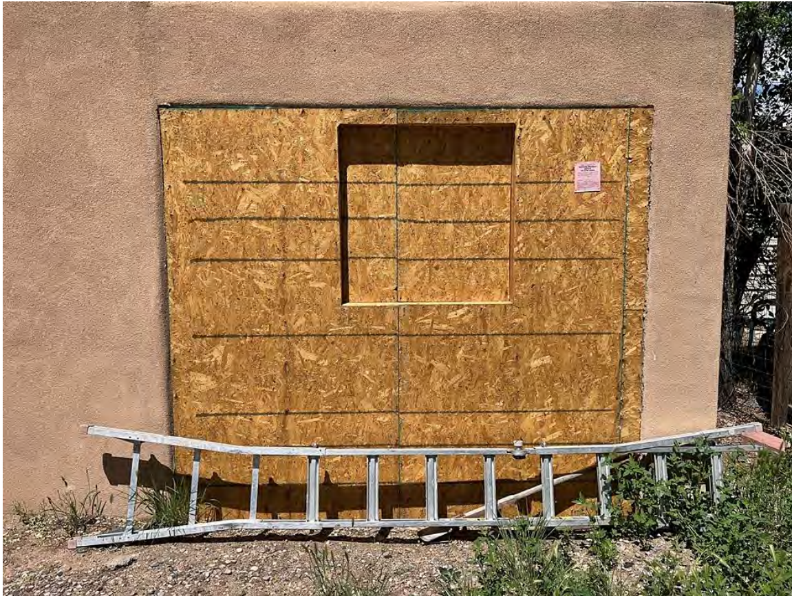
Photo 35: Infilled garage door. Camera facing west.
