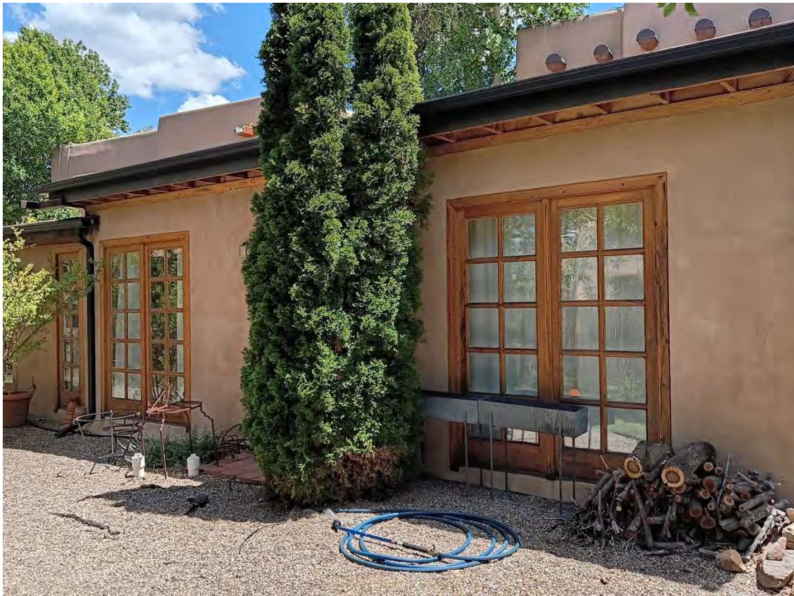
Photo 10: North elevation, east end. Camera facing southeast.
