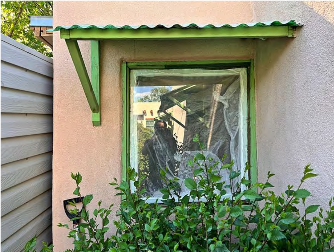
Photo 8: Window at CMU addition. Camera facing west.
