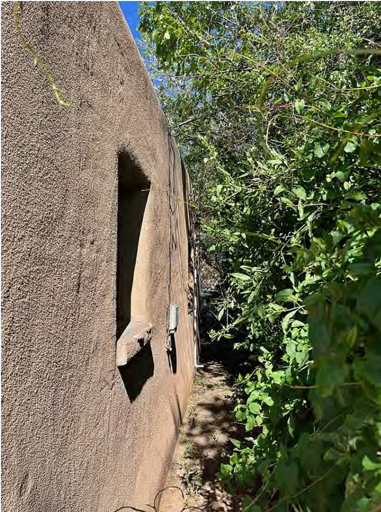
Photo 43: South elevation. Camera facing east.
