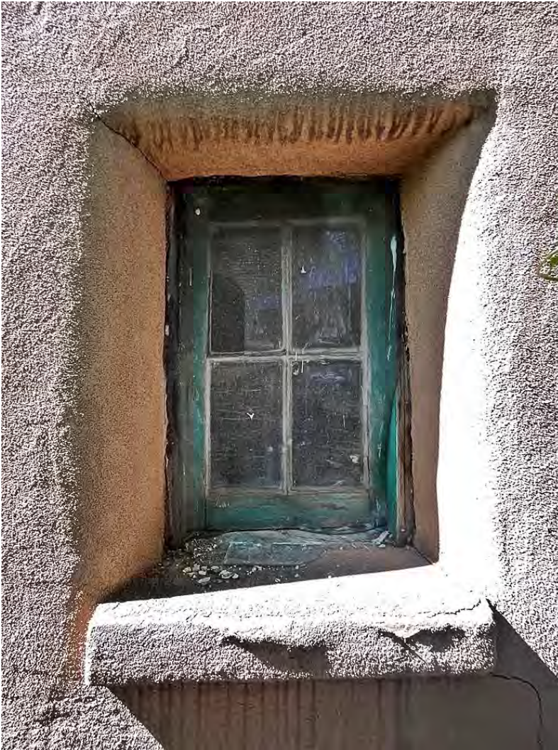
Photo 44: West end window. Camera facing north.
