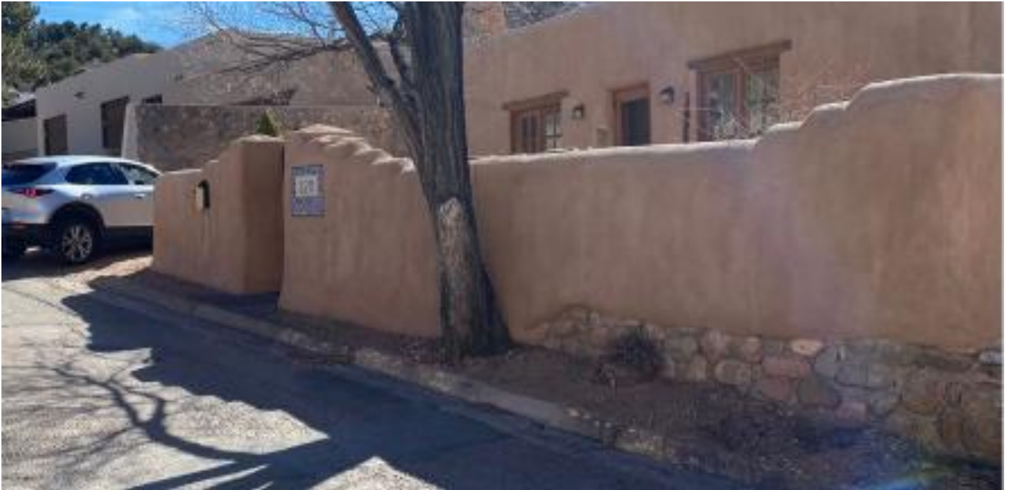
Figure 5: East Property Line Yard Wall
