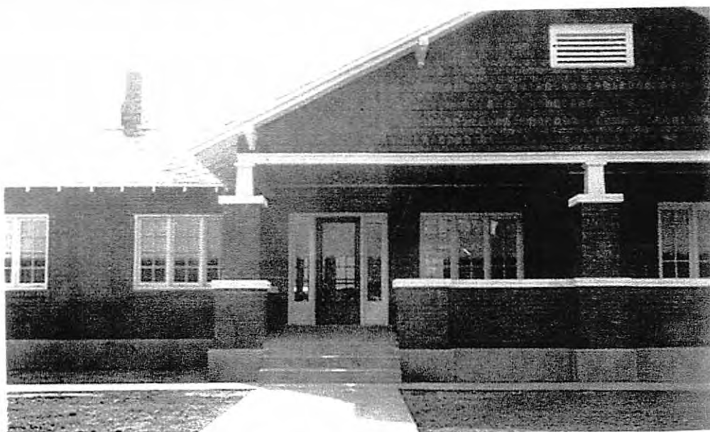
east, front elevation of one story brick bungalow
