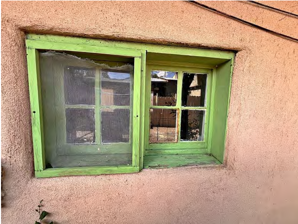
Photo 27: Window at apartment kitchen. Camera facing north.
