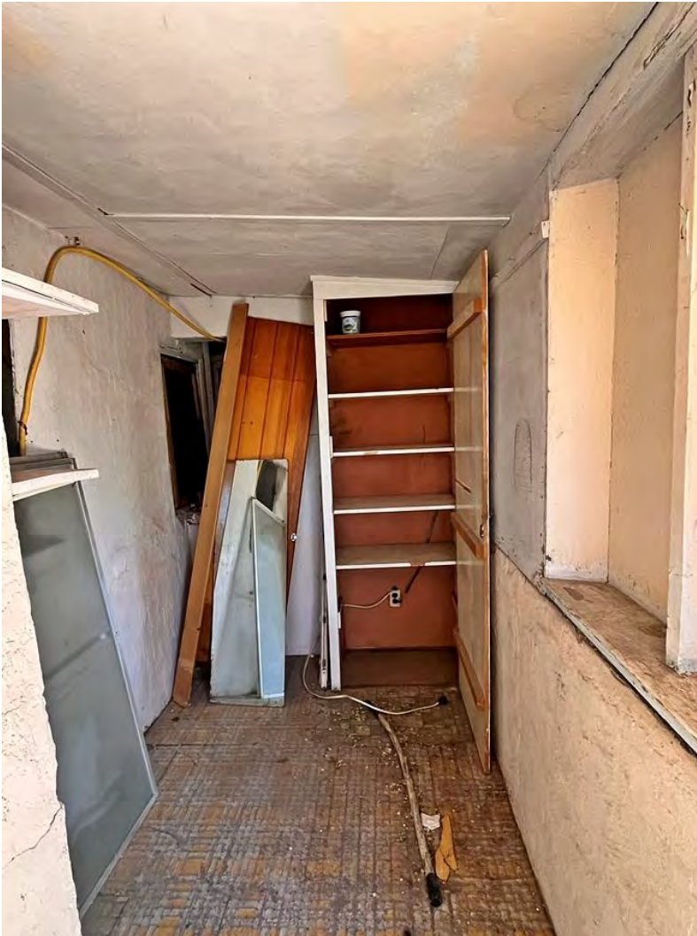
Photo 14: Interior of enclosed porch. Camera facing south.
