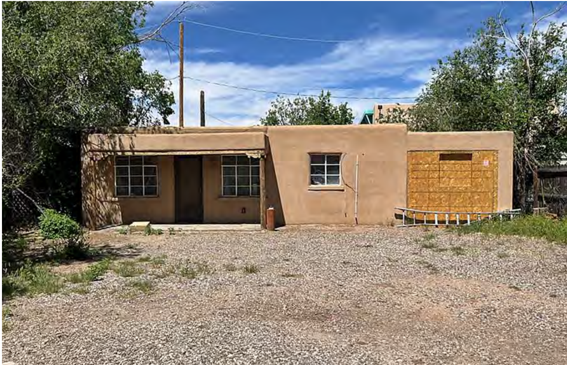
Photo 29: East façade and context. Camera facing west.
