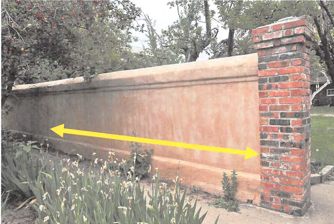
Figure 6: Section of reconstructed wall along West Santa Fe Avenue, as per Peter Komis and visual evidence.
