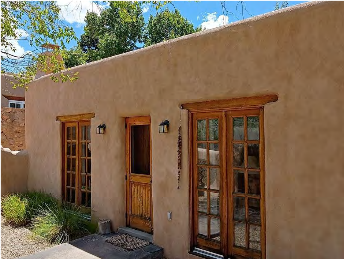
Photo 3: East (front) façade. Camera facing southeast.
