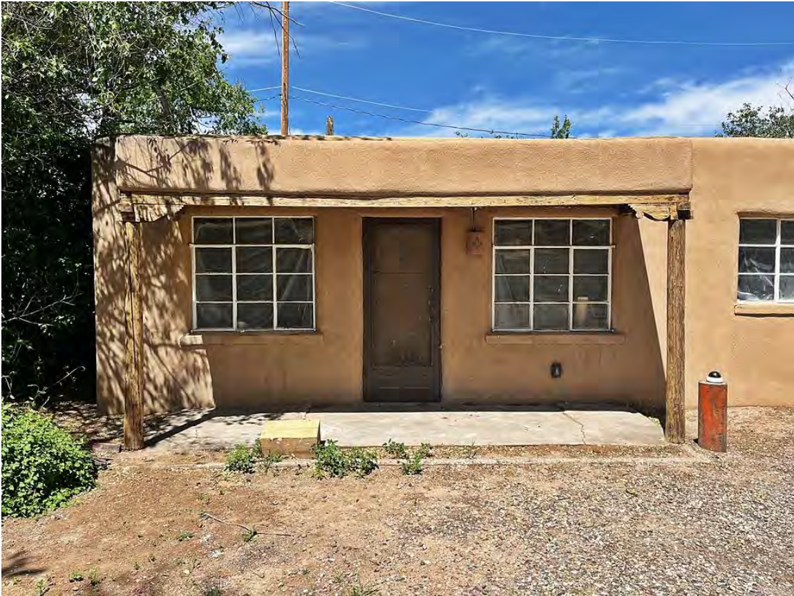
Photo 30: Porch. Camera facing west.
