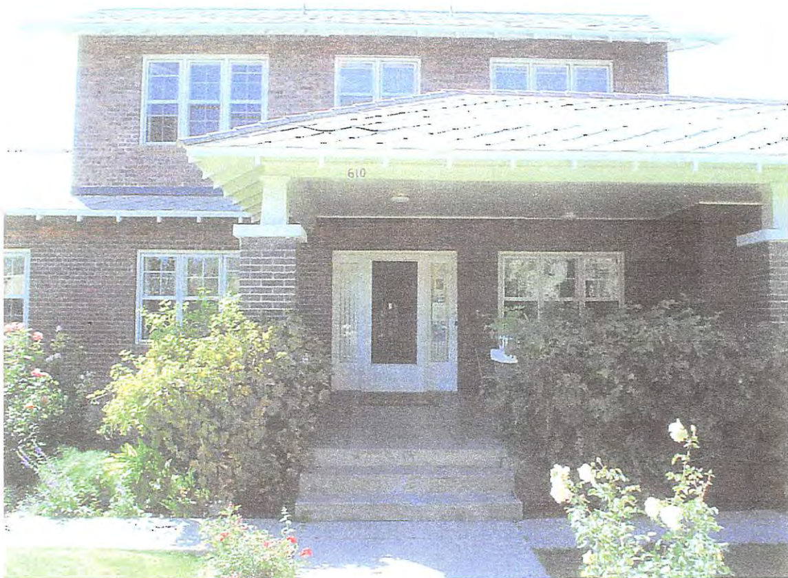
Front Entrance, East Elevation
