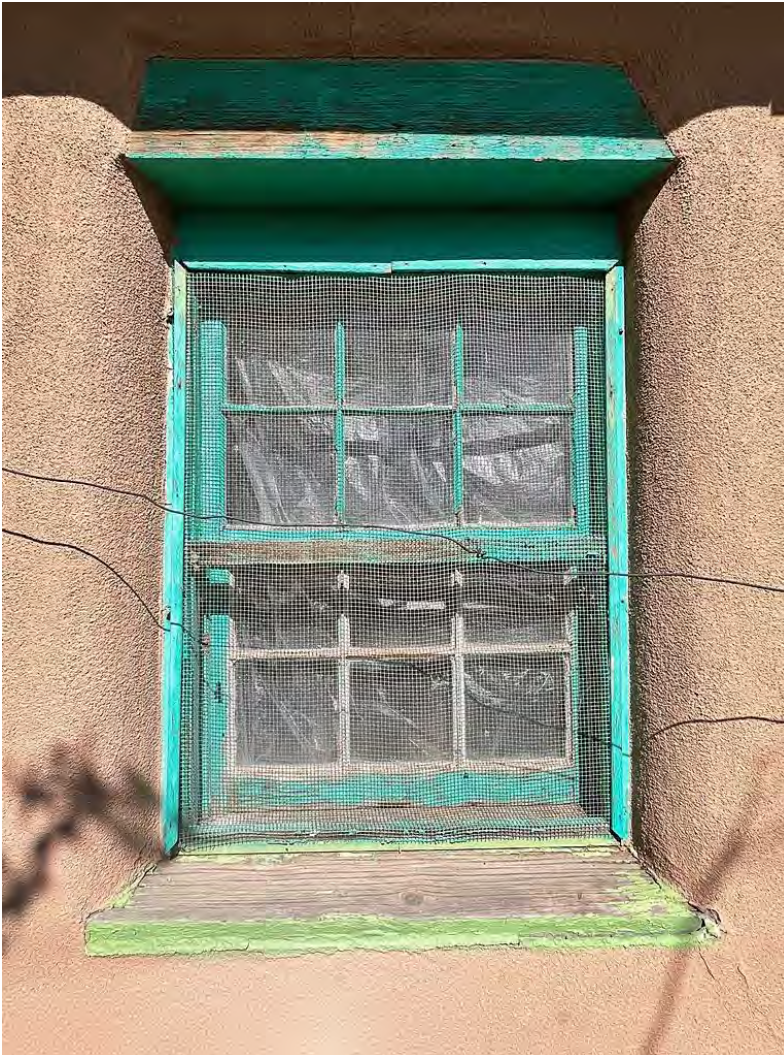
Photo 42: Window south of door. Camera facing east.
