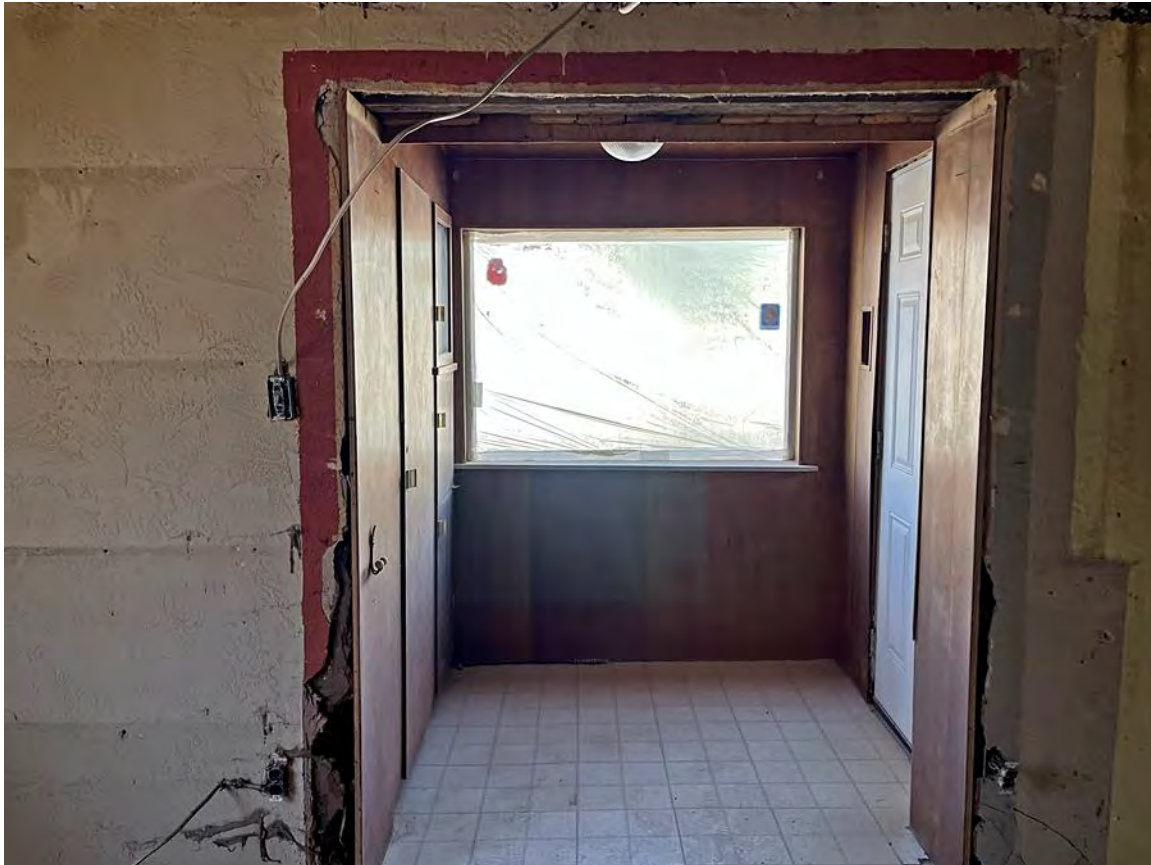
Photo 6: Entry vestibule. Camera facing east.
