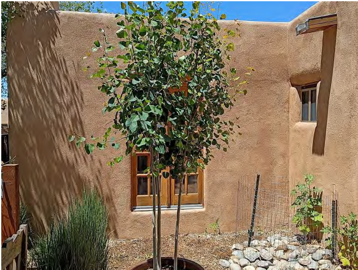
Photo 5: South elevation, west end. Camera facing north.
