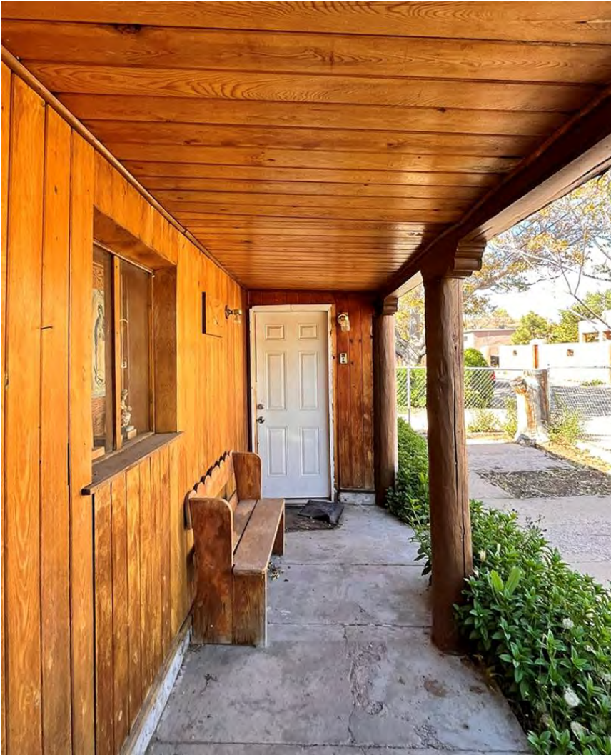
Photo 3: Portal and entry vestibule. Camera facing north.
