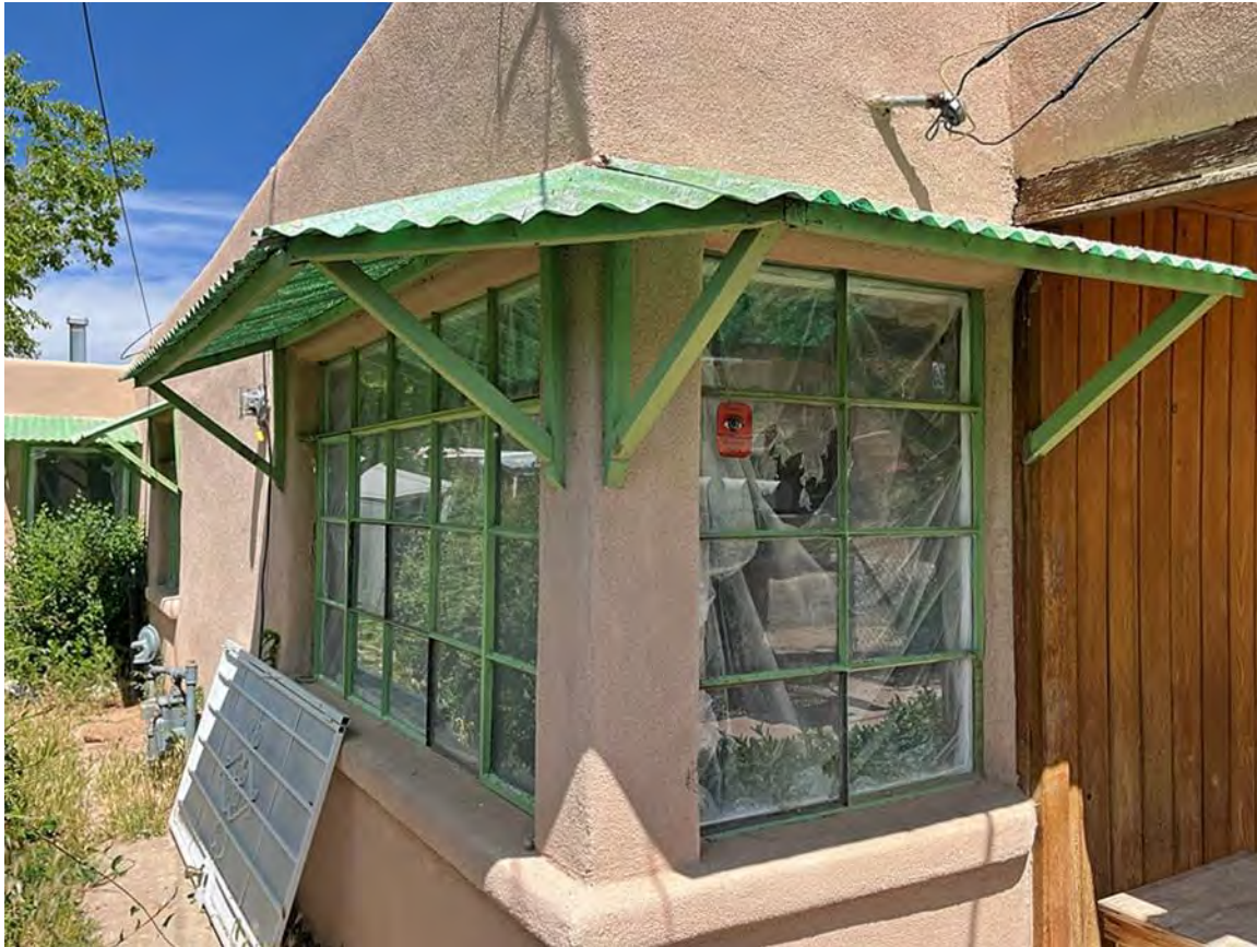
Photo 7: Windows at southeast corner. Camera facing northwest.
