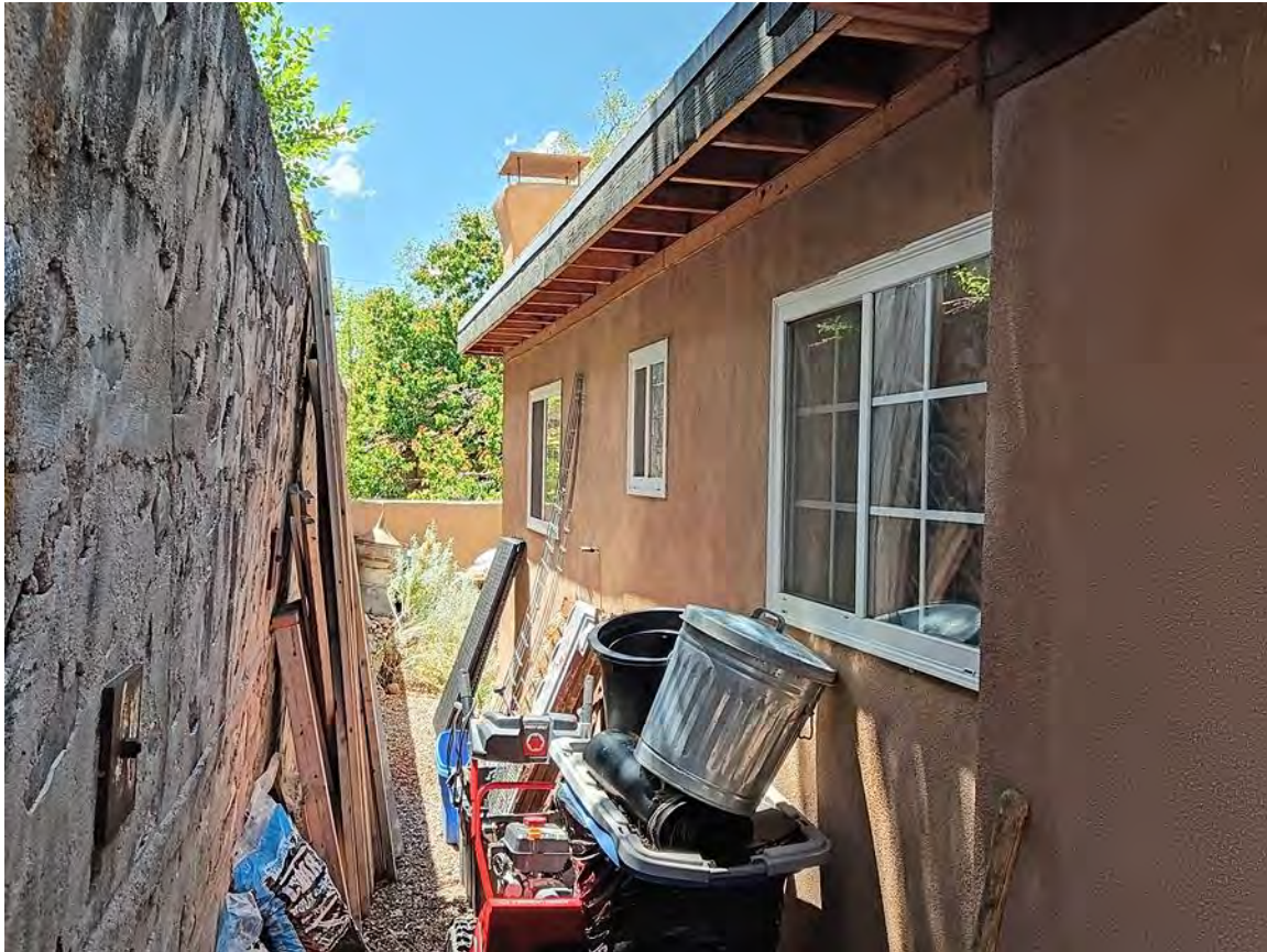
Photo 13: South elevation, west end. Camera facing west.
