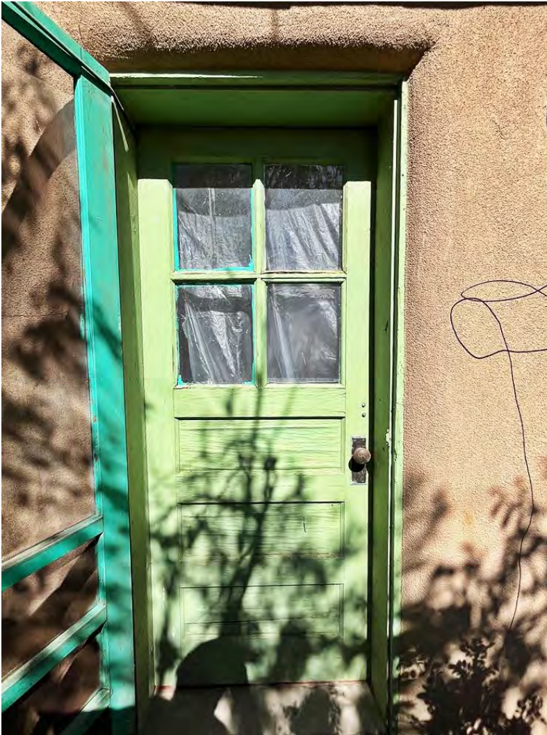
Photo 40: Rear entry door. Camera facing east.
