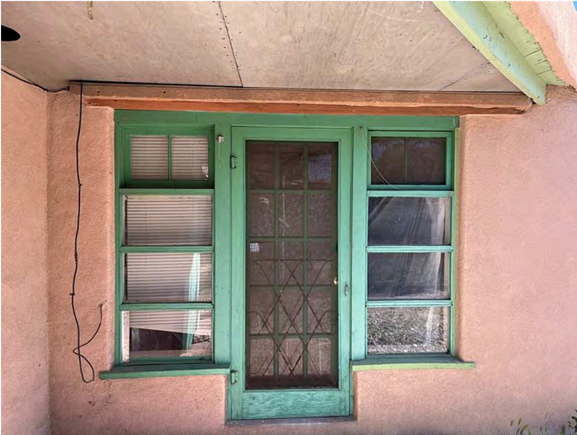
Photo 15: Entry to CMU addition. Camera facing south.
