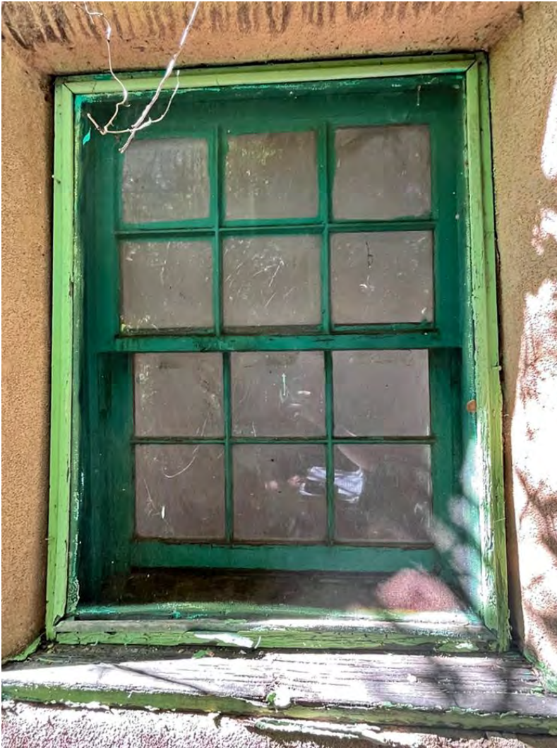
Photo 45: East end window. Camera facing north.
