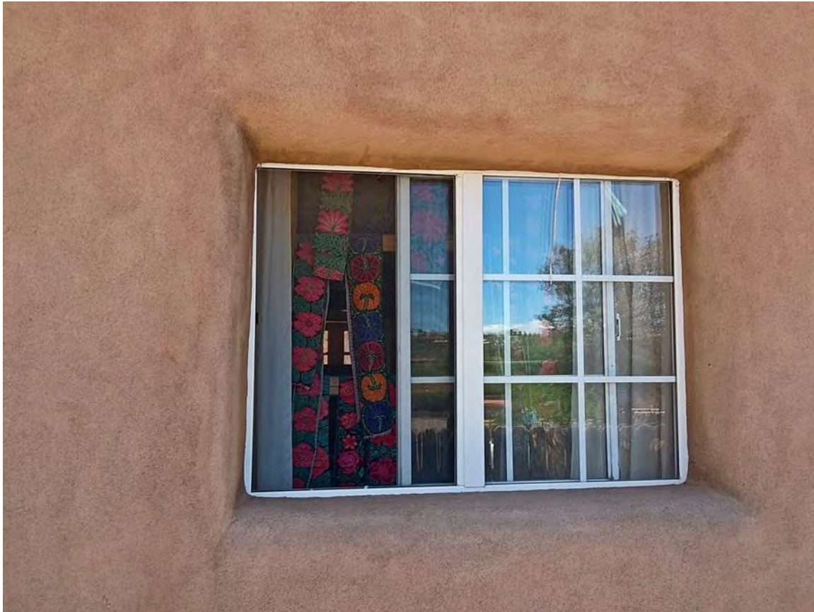
Photo 8: North elevation. Window detail. Camera facing south.
