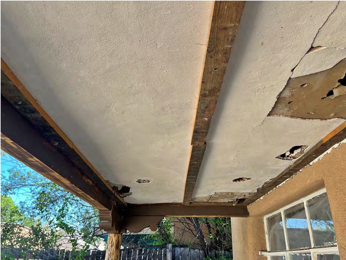
Photo 31: Porch ceiling. Camera facing up.
