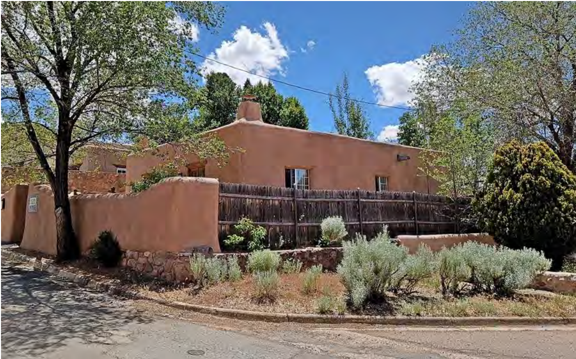
Photo 2: Setting and east and north elevations. Camera facing south.
