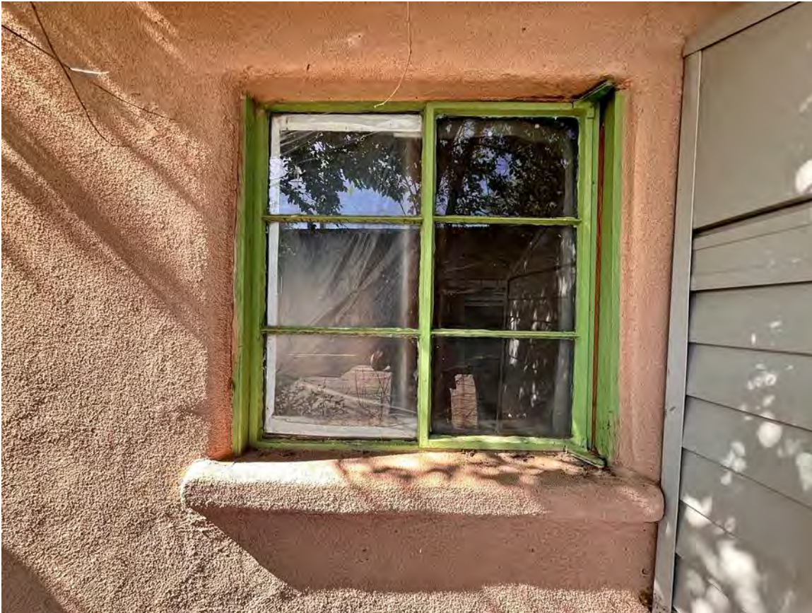
Photo 25: Window at CMU addition. Camera facing north.
