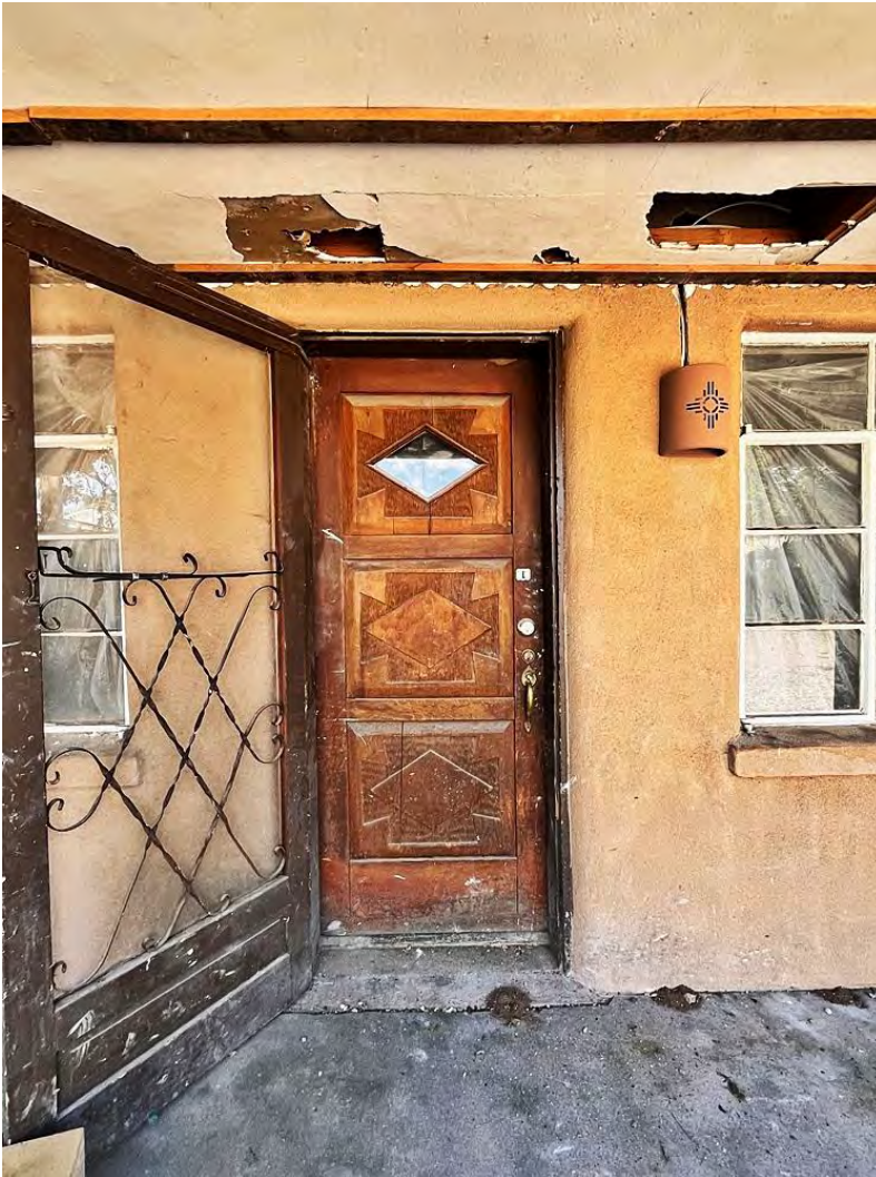
Photo 32: Entry door. Camera facing west.
