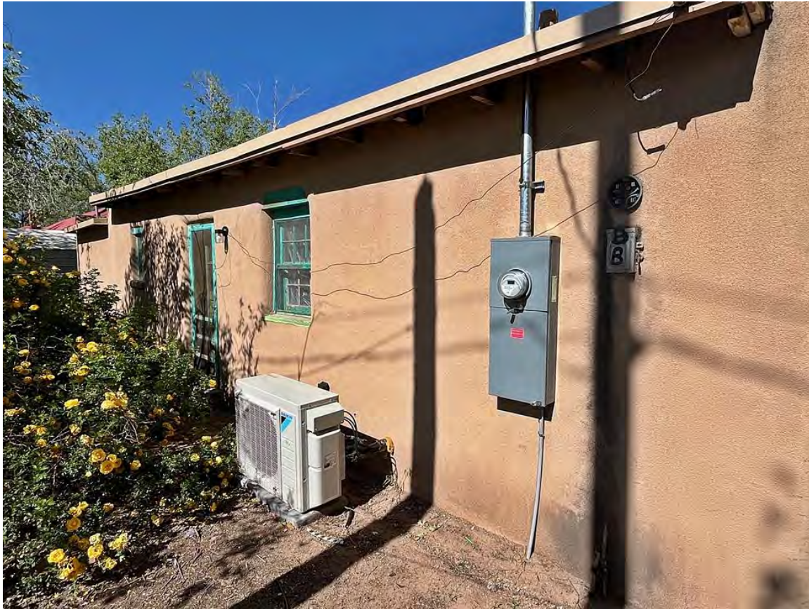
Photo 39: West elevation. Camera facing northeast.
