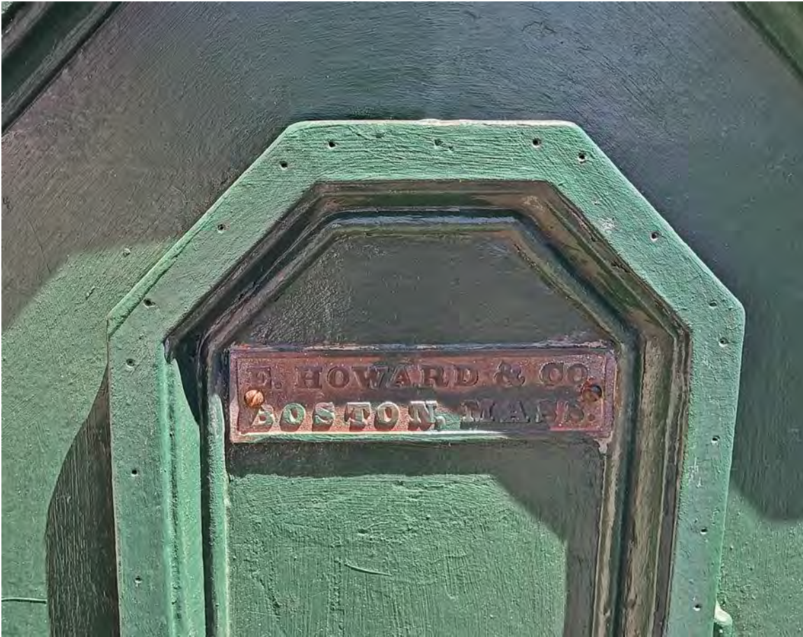
Photo 5: Base at west elevation, manufacturing nameplate. Camera facing east.
