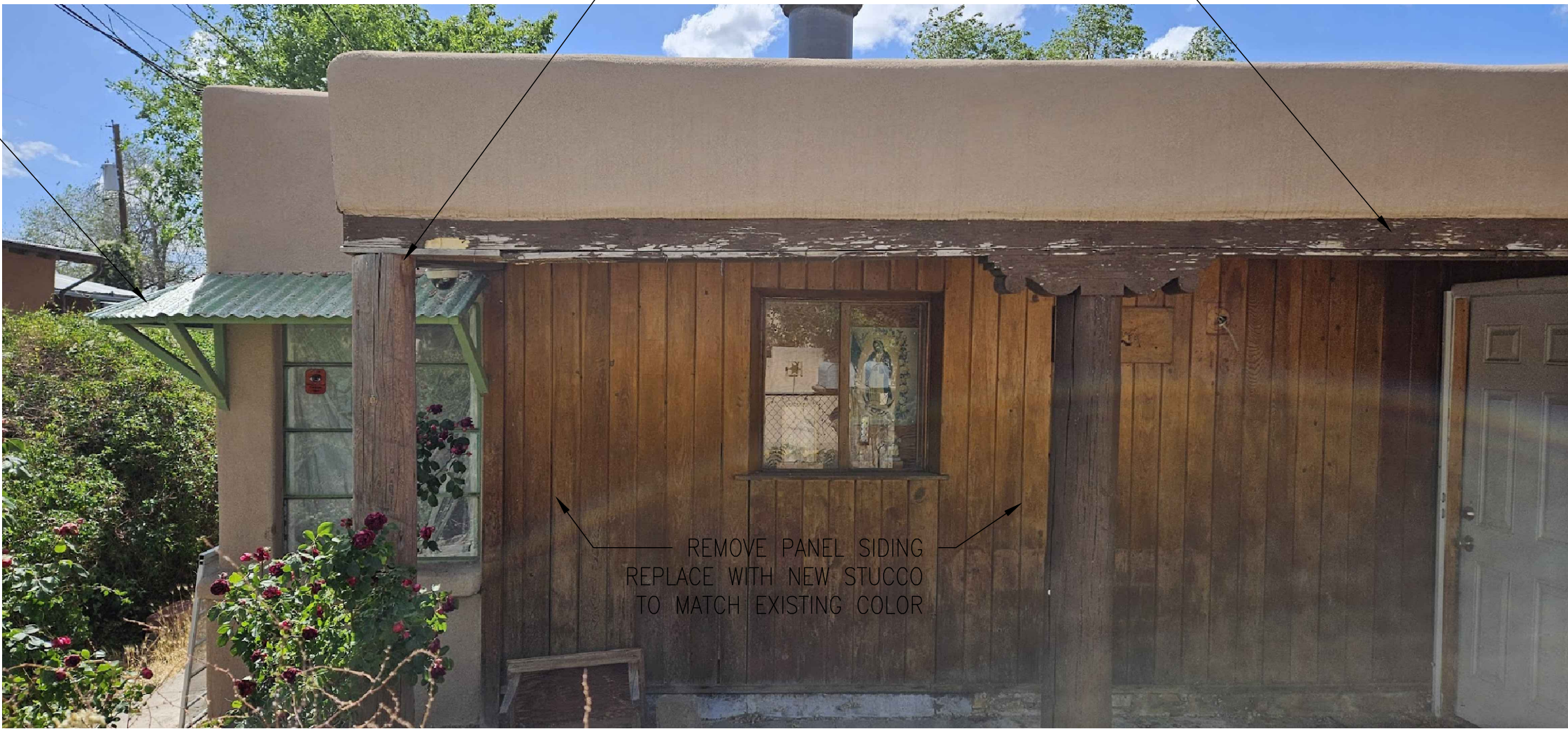
EXISTING EAST ELEVATION (FRONT)
