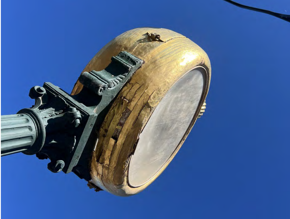
Photo 11. Detail of damage to clock face, view looking up from northeast corner. (July 2026)
