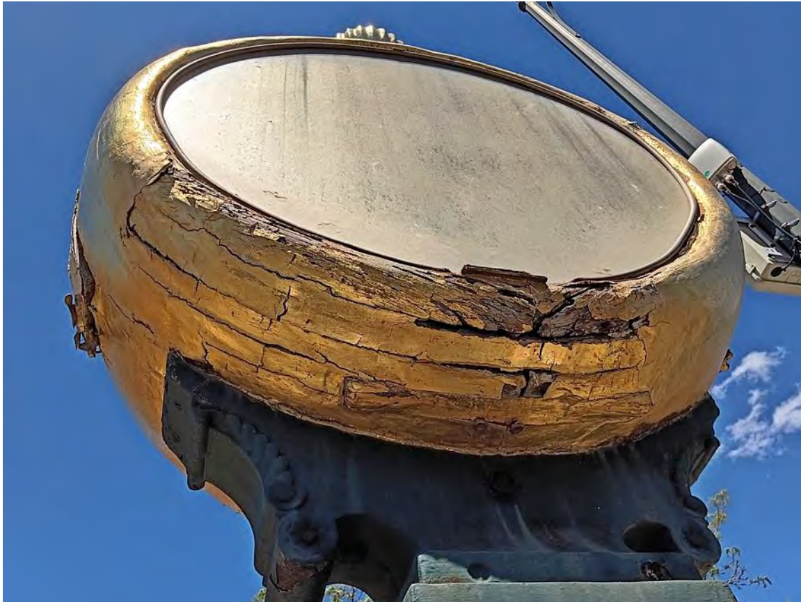
Photo 10: South elevation head: bracket, casing, and Plexiglas dial. Camera facing up.
