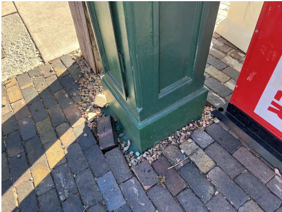
Photo 18. Brick pavers and gravel infill surrounding Spitz Clock and historic plaque, view looking down from southwest corner. (July 2026)
