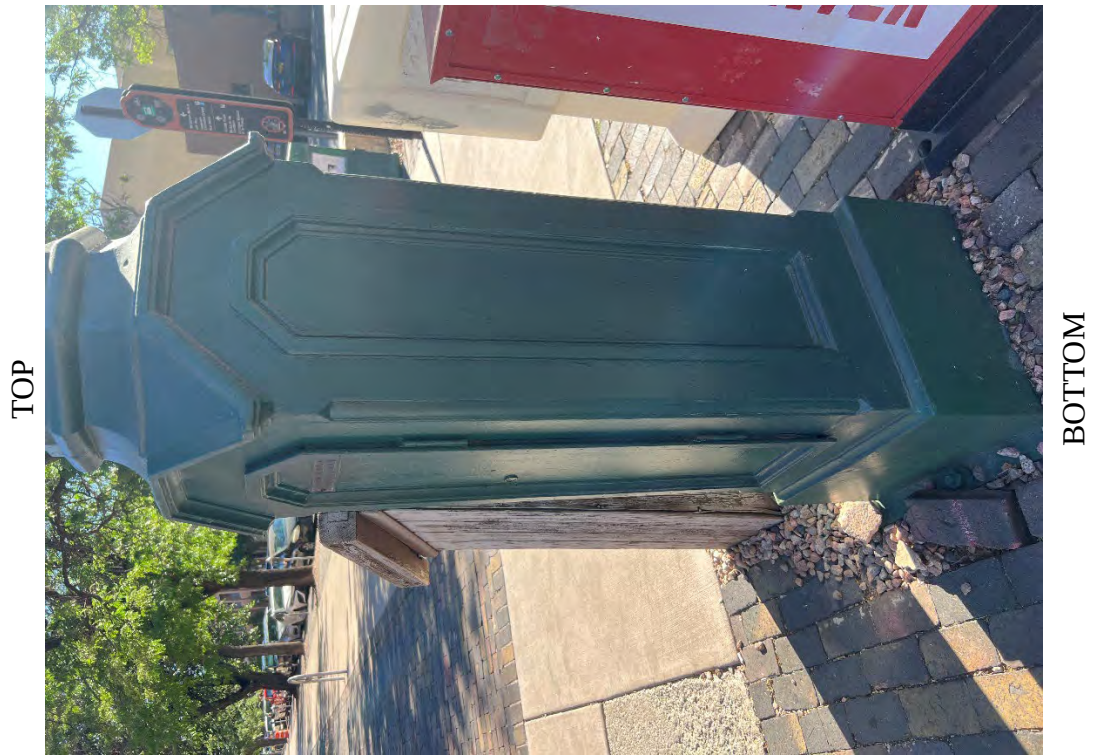
Photo 7. Spitz Clock south and east base detail, view northwest. (July 2026)
