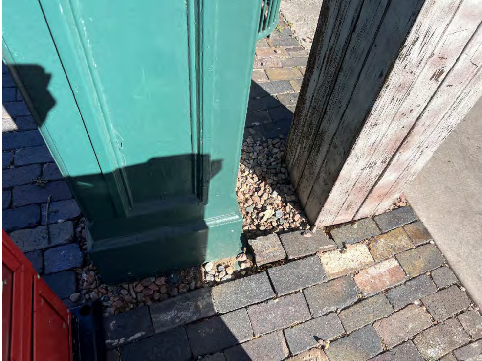
Photo 17. Brick pavers and gravel infill surrounding Spitz Clock and historic plaque, view looking down from east elevation. (July 2026)
