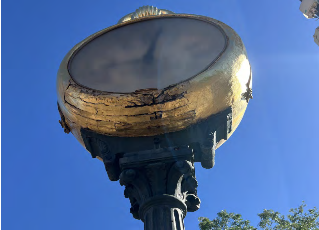
Photo 9. Detail of south face casing, view looking up. (July 2026)
