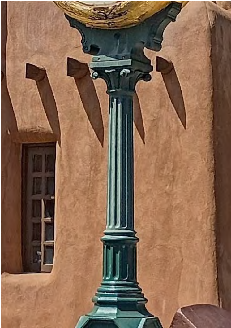
Photo 6: Shaft, capital, and bracket. Camera facing northwest.
