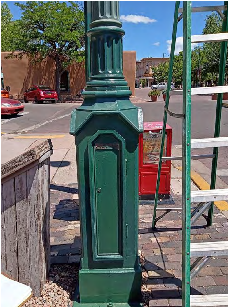
Photo 4: Base at west elevation, winding access door. Camera facing east.
