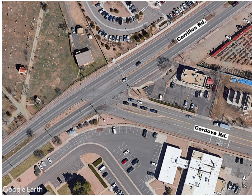
Figure 13 - Aerial Image: Intersection #2
