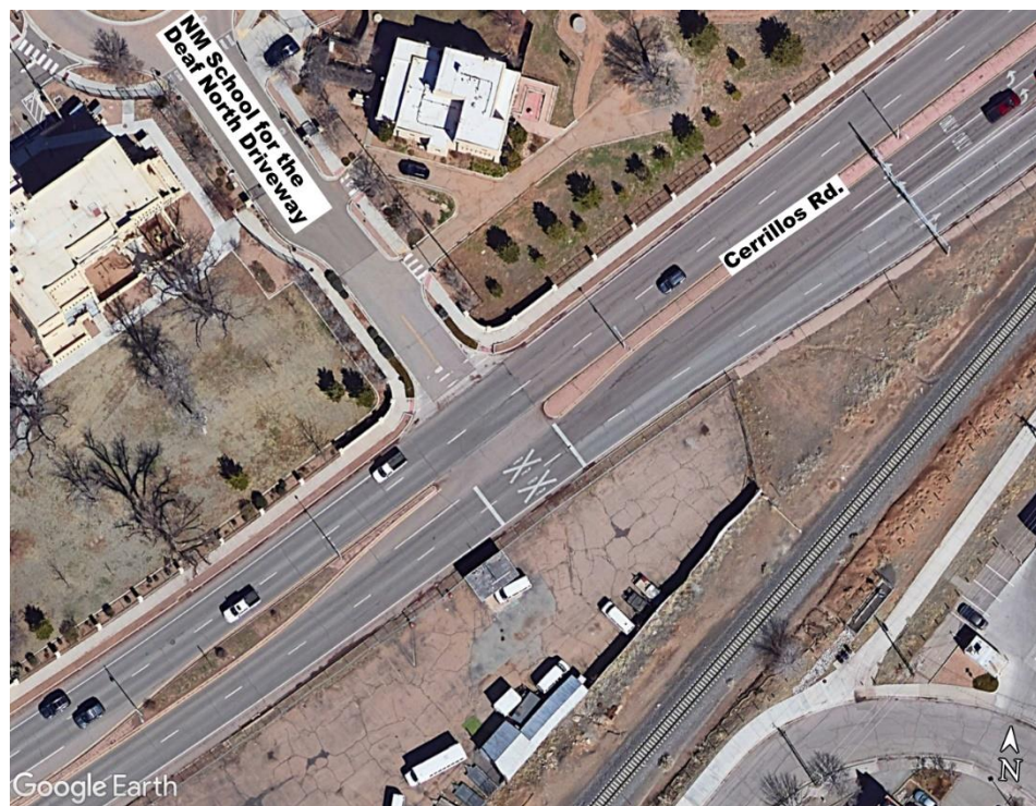
Figure 14 - Aerial Image: Intersection #3
