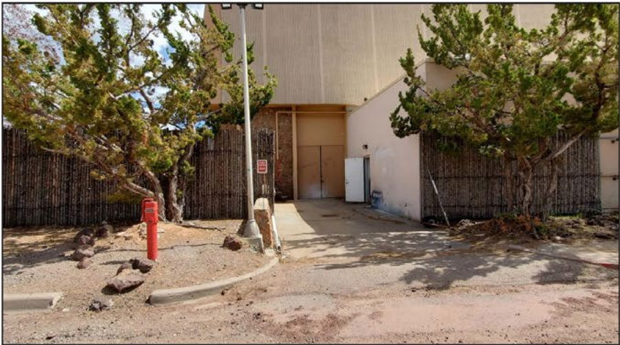
4) View of loading area
