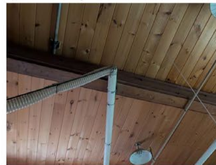
6) Metal Bracing in Shop
