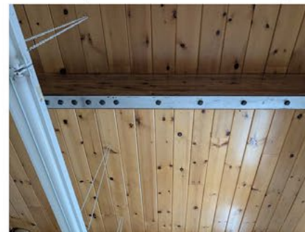
4) Metal Bracing in Classrooms
