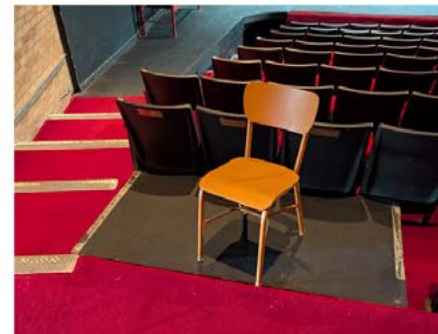
2) Auditorium Wheelchair Area
