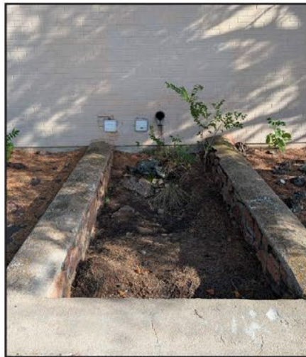
3) Roof Water Catchment Area
