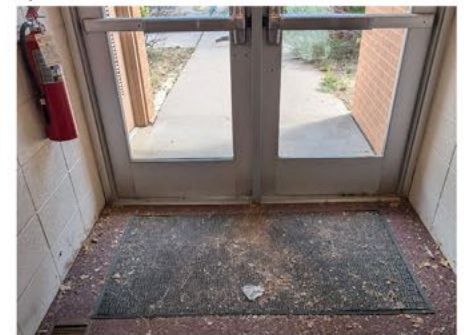
6) Exit Doors in Corridor 115
